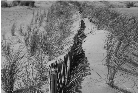
Fig. 6 - Reed sand fences create accretion zones upwind, and shadow areas of sand deposition downwind, but this rule only works when the orientation of the sand fence is properly located perpendicular to the prevailing wind. Taller sand fences are more visually intrusive and their effectiveness is restricted to the narrow upwind strip and the “shadow” area which width is no longer than 3 or 4 times the height of the fence.
