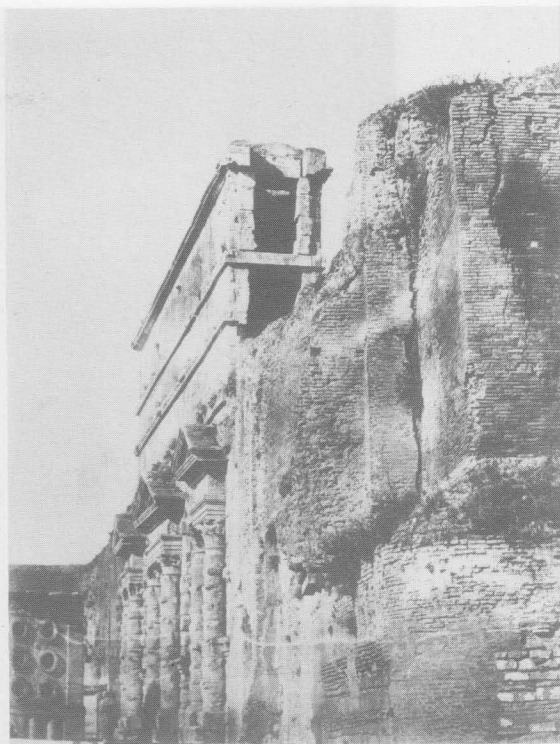
Fig. 3 - The Porta Maggiore was the gate to the road to Praeneste (modern-day Palestrina). The gate supported a tract of the Claudian aqueduct. The photos taken in 1864-66 show the walls covered by a rich vegetation composed mostly of Rubus bushes, fig-shrubs and in the fissures Parietaria , Cymbalaria , Asplenium , etc., and many caper-bushes of which the 'fruits' (the buds) has been harvested.
